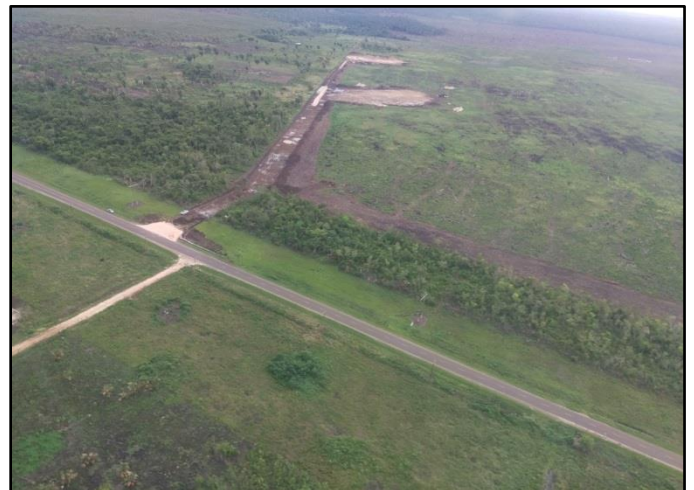
Northerly view of new access road/EPZ – June 15 th 2015
